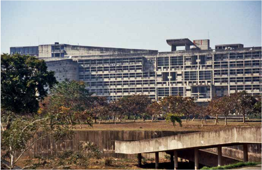
fig. XXV: The ten-storied Secretariat is the tallest structure of Le Corbusier's Capital Complex.
