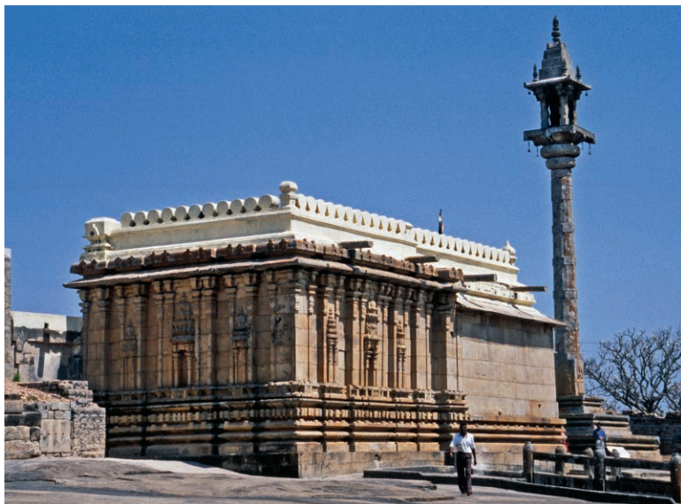
Plate 10: The Antarāla Pārśvanātha Basadi on Candragiri is a late Hoysala construction, the front hall of which illustrates a tendency towards a return to greater simplicity in later structures.
